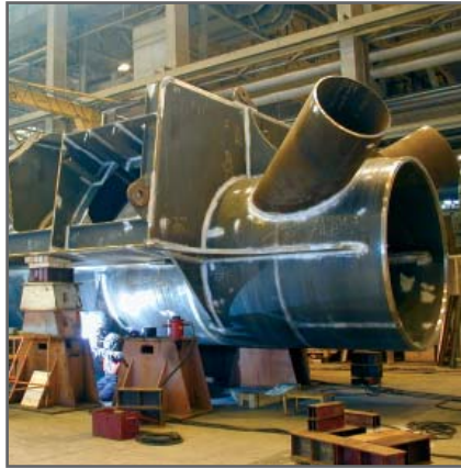
Welding of truss connection for spar hull
