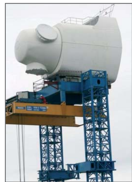
Installation of wind power unit in the field
